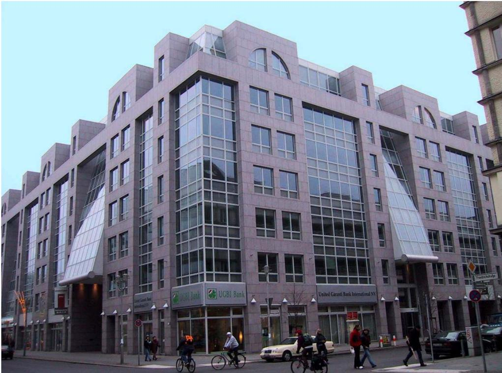
PREFABRICATED UNITIZED FACADE WITH SLOPED GLAZING 9° AND 13°
