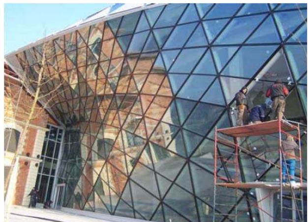
CONSTRUCTION: FREE SPAN MAIN STEEL WITH ROUND TUBES IN FORM OF A WHALE
