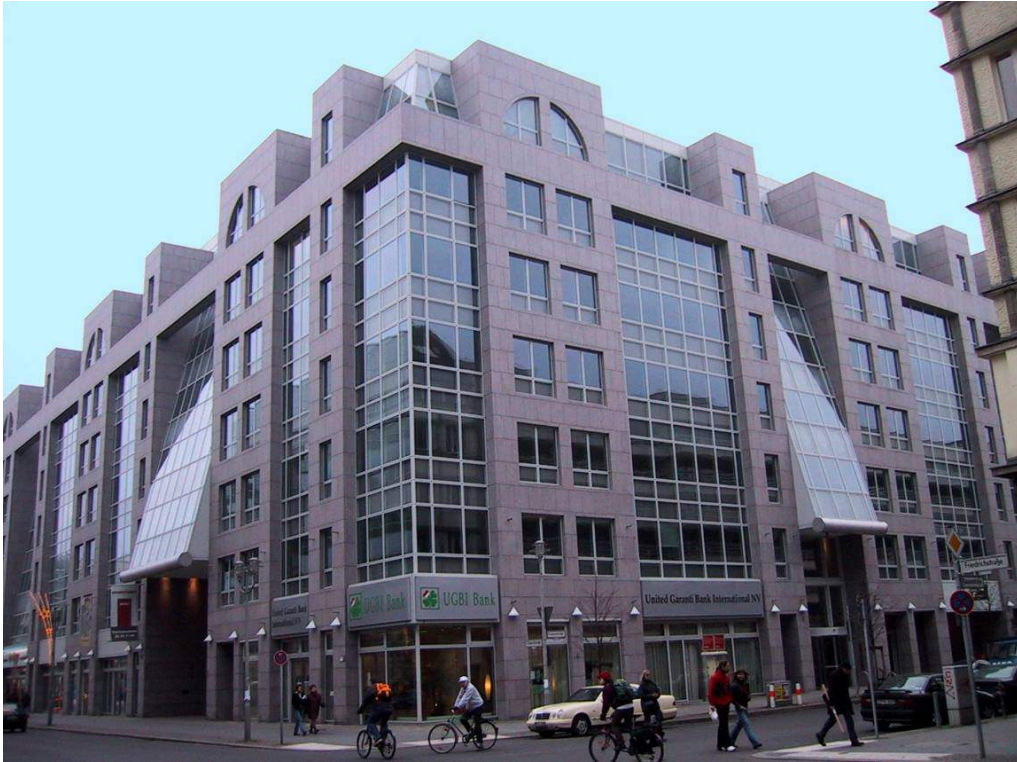
PREFABRICATED UNITIZED FACADE WITH SLOPED GLAZING 9° AND 13°
