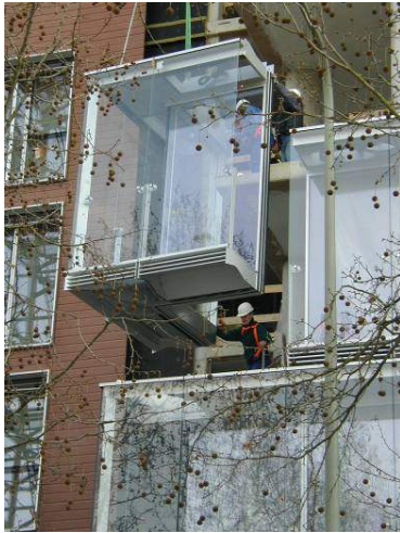
HOOKING CORNER ELEMENT AT TOWER
