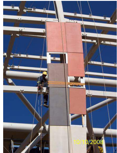
WORK AT SPECIAL ELEMENTS
