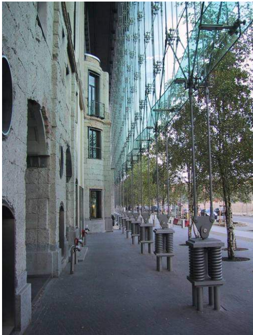
ANCHOR CABLE WITH GLASSCREEN/OLD BUILDING
