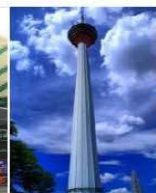
TELECOM TOWER KL
