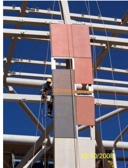
WORK AT SPECIAL ELEMENTS
