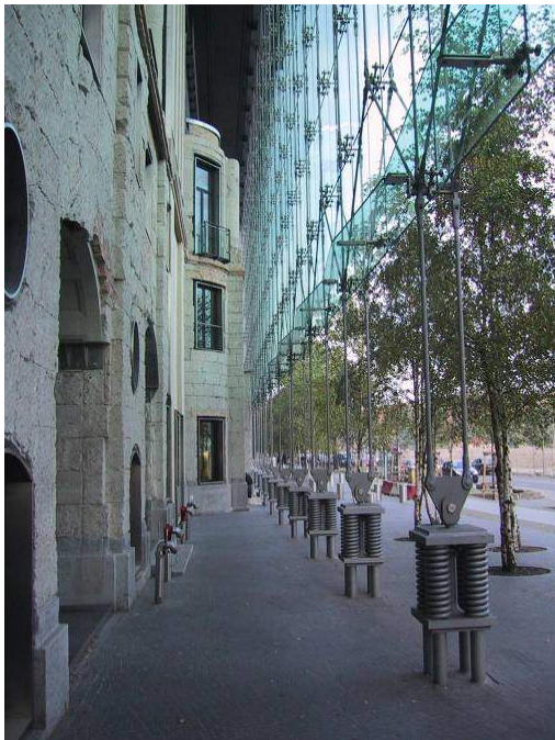
ANCHOR CABLE WITH GLASSCREEN/OLD BUILDING
