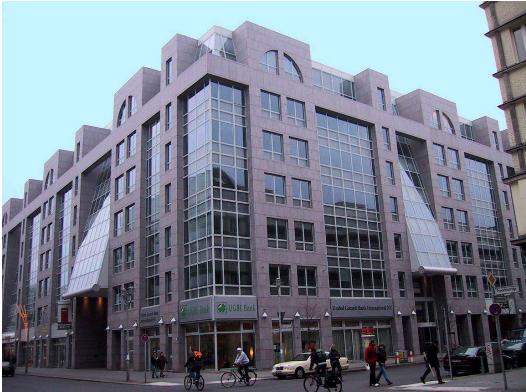
PREFABRICATED UNITIZED FACADE WITH SLOPED GLAZING 9° AND 13°
