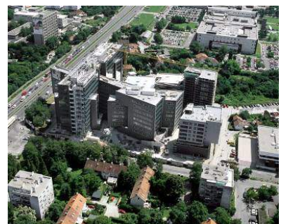
OVERVIEW OF THE AREA
