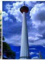
TELECOM TOWER KL
