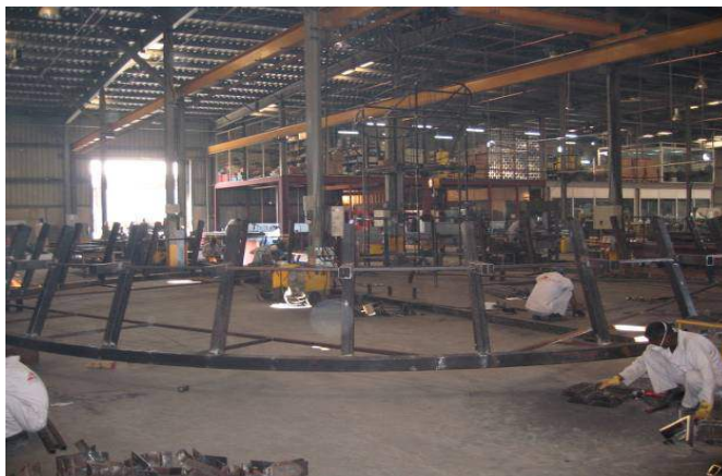
STEEL PRODUCTION AT WORKSHOP
